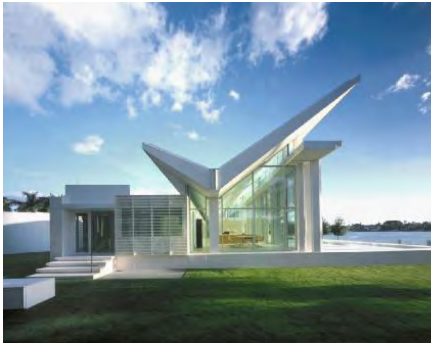
Neugebauer House . Naples, Florida. 1995-1998. ©Richard Meier & Partners/ESTO Photographics
